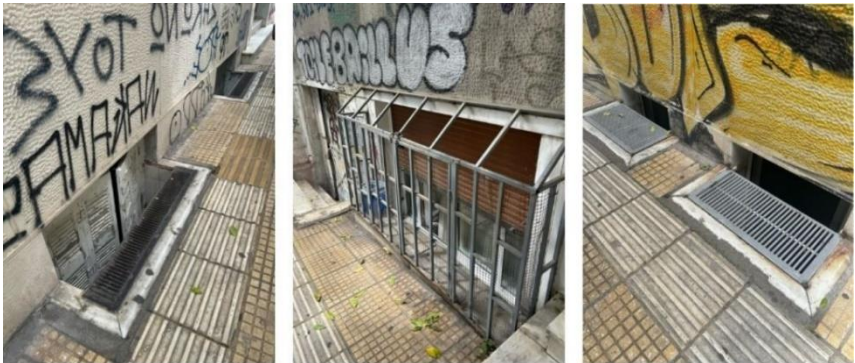
Picture 4, 5 & 6: Basement apartments' view from the sidewalk
